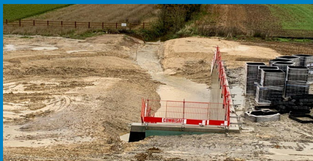
River Ash flowing into the new culvert during a storm
