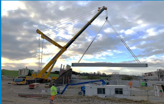
One of five beams being lifted into place at the River Ash
