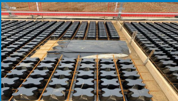
Above and below image: Grasscrete installation at Lloyd Taylor Drain
