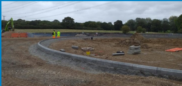
Kerbs being laid for Hadham Park roundabout
