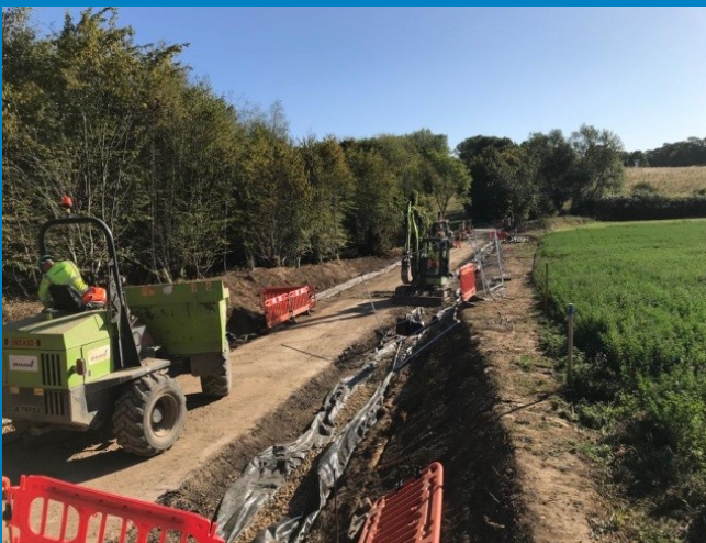
Road reconstruction at Upwick Green
