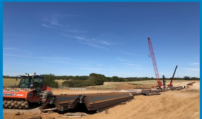
Sheet Metal Piling at Albury Tributary
